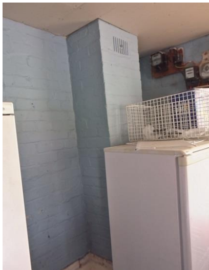
Fig 15 and 16: inside the cookhouse showing the chimney breast with air vent and blocked up stove pipe entrance. A boiler or stove was located here with a water tank above in the roof space.
