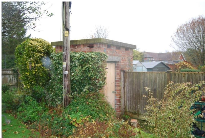
Fig 17: Pumping station showing the ventilation gaps just under the concrete roof.
