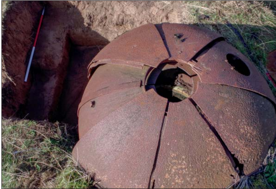
Plate 17: Top view of the steel dome structure, showing overlapping steel plates, double skin and other fittings. Looking west
